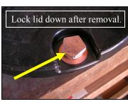
a 1" socket, a vice-grip type or slip-joint pliers can turn the 5-sided lid locking device. Something placed over the meter in the winter protects the meter from freezing and locates it clearly. A simple electric fence post might be used if you don't place protection over the pit in cold weather.
